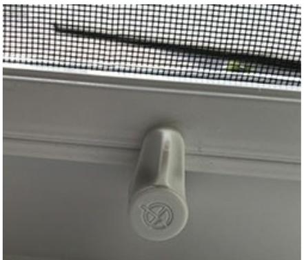
5. Once the screen has been hung in position secure the turn buttons in place to hold the fly screen panel closed.
