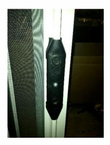
The shoot bolt is hidden behind the handle assembly and is operated by squeezing the centre handle buttons together to retract the bolt and releasing to engage the bolts into the holding catches.
